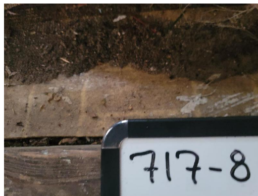
717-8 Rolled Flooring/Adhesive Interior Southeast Bedroom
