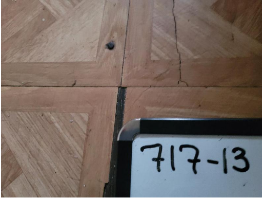
717-13 12"x12" Floor Tile/Adhesive Interior South Bathroom
