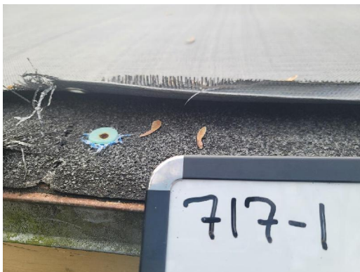
717-1 Rolled Asphalt Roofing/Tar Typical Exterior Roof
