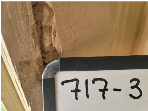
717-3 Drywall/Joint Compound Typical Interior Walls/Ceilings
